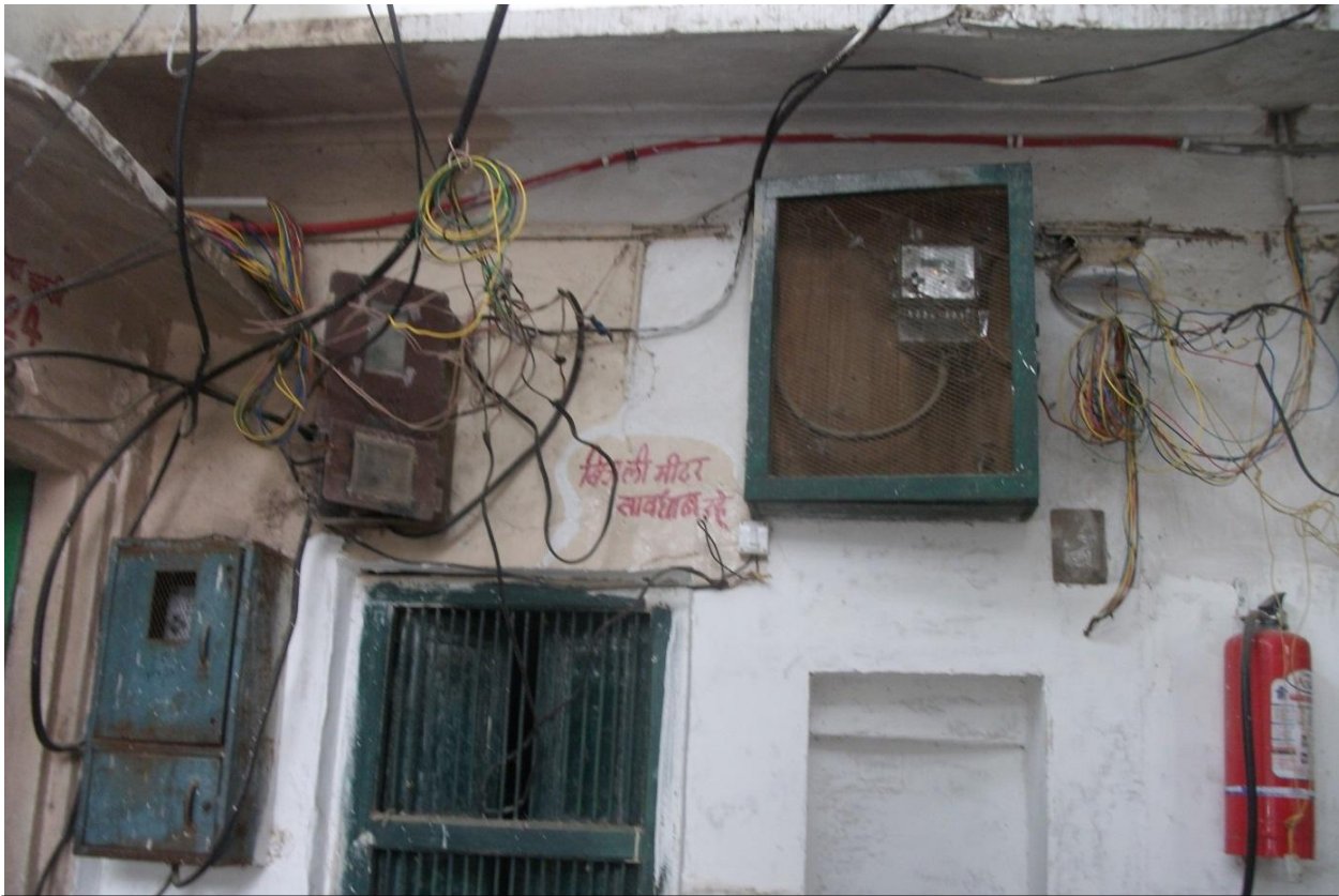
Image 10.44: Haphazard wiring (Source: SHC)
