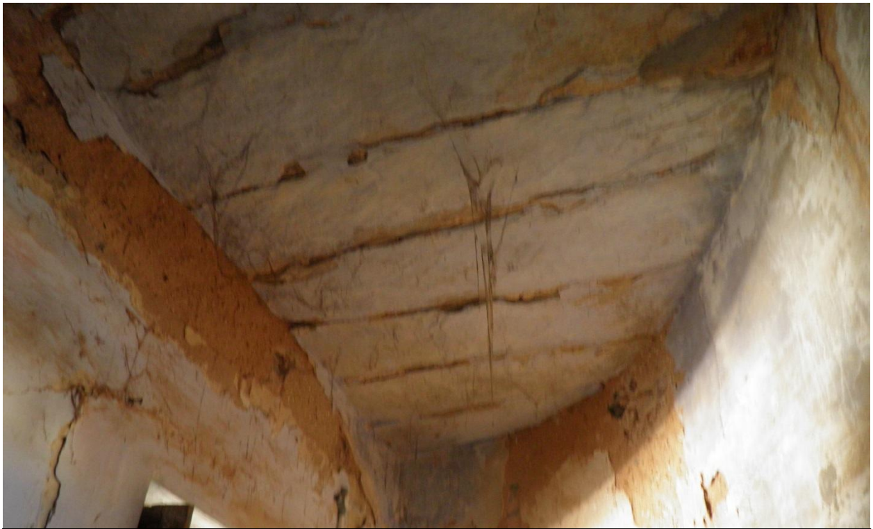
Image 10.30: Cracks visible in the bastion (Source: SHC)
