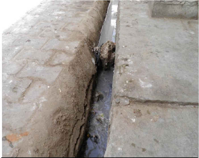
Image 8.4: Stone Stuck in open Drainage system (Source: SHC)
