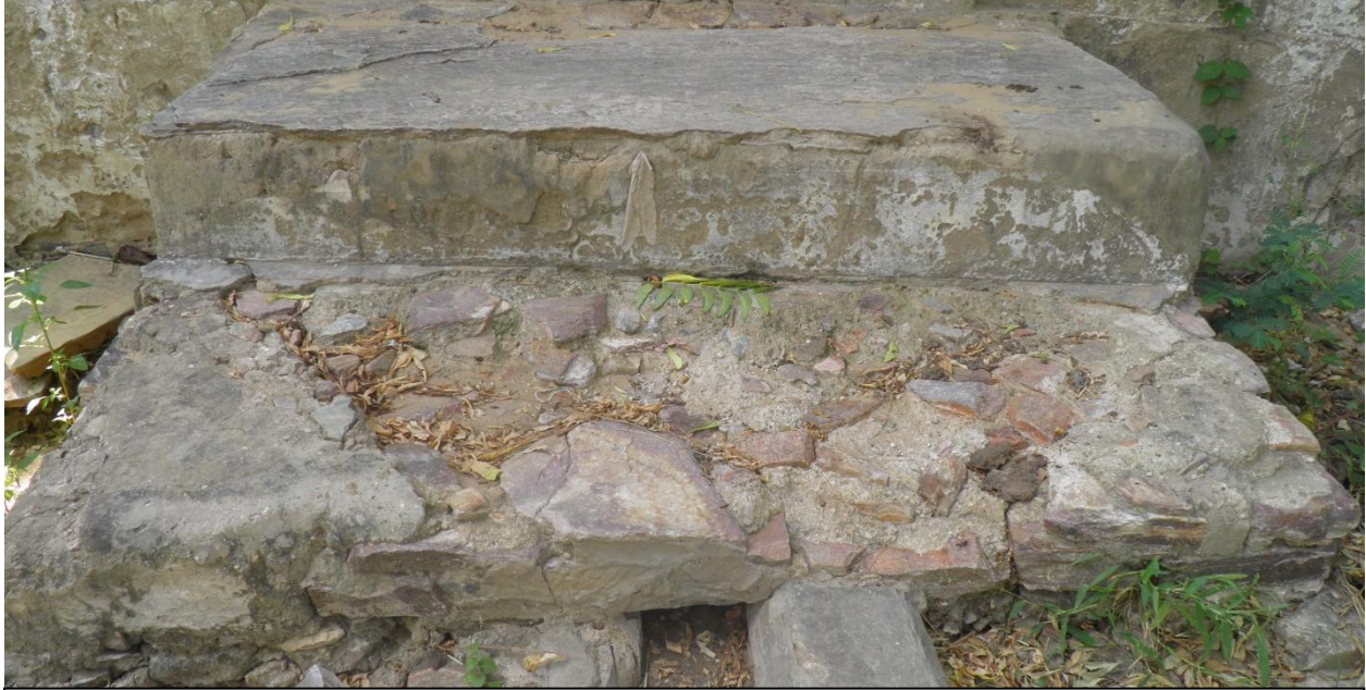
Image 10.43: Broken steps making the accessibility difficult (Source: SHC)
