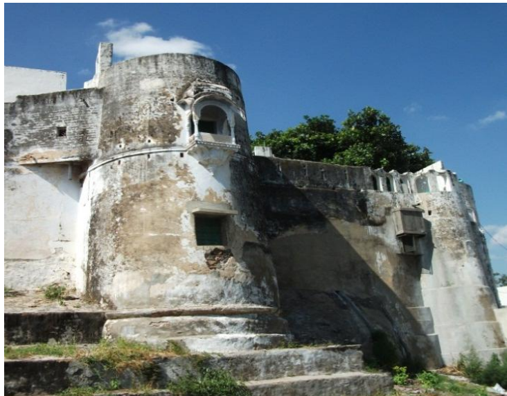
Image 10.11: Massive tapered buttressed walls, interrupted by bastions (Source: SHC)
