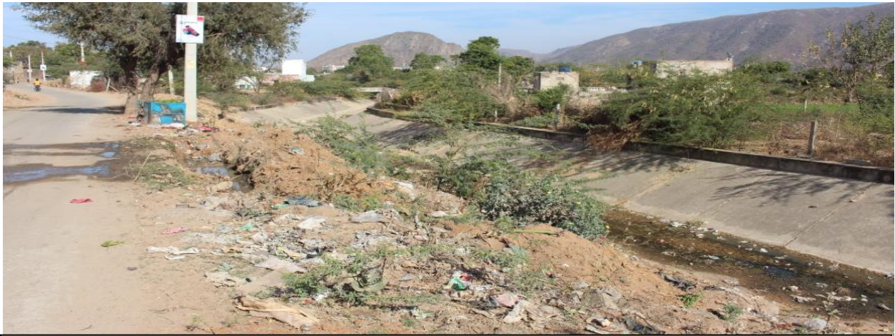
Image 12.18: Image showing drains overflowing into the feeders (Source: SHC)
