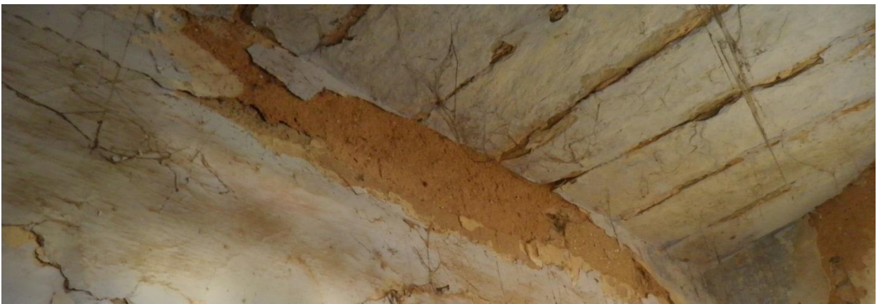
Image 10.32: Flaking of plaster in Bastion (Source: SHC)
