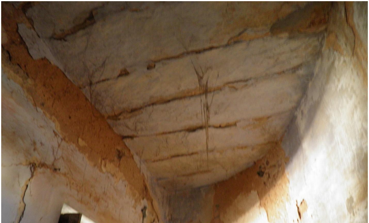
Image 10.30: Cracks visible in the bastion (Source: SHC)
