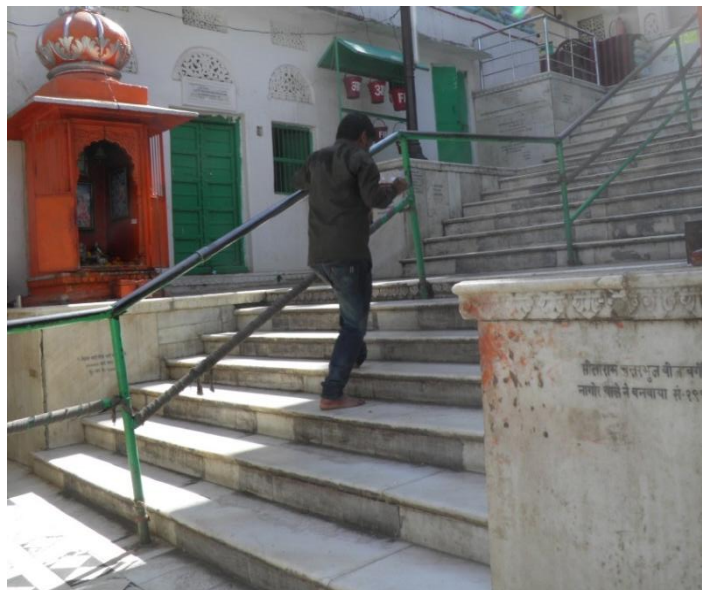
Image 10.57: No provision of lifts or ramps. (Source: SHC)
