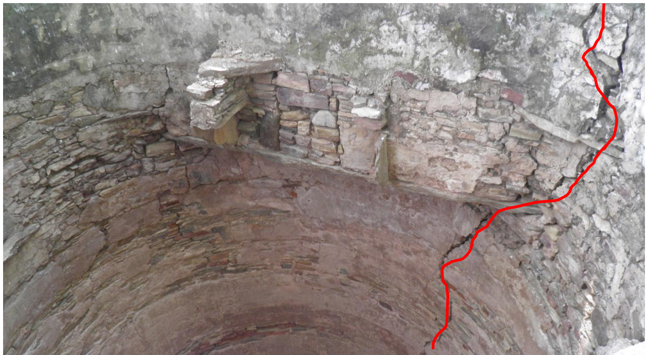
Image 10.42: Cracks inside well (Source: SHC)
