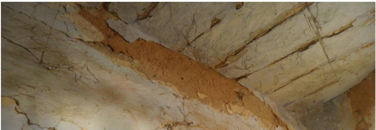
Image 10.32: Flaking of plaster in Bastion (Source: SHC)
