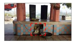
Condition C4 - Incompatible additions in Cement Concrete over local stone
