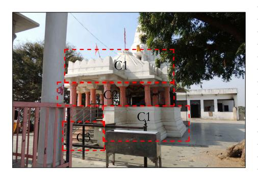
Condition C1 - Incompatible Addition - Cement Paint over Original Stone, C2 - Incompatible Intervention -Oil Paint over Original Stone, and C3 - Incompatible Later Intervention/ Addition - Kota Stone over Original Stone
