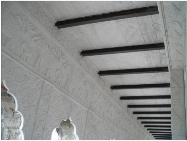
Image 3 Marble & I-sections in the ceiling
