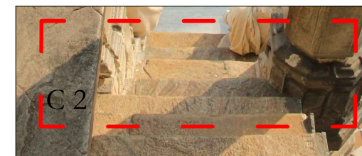
C 2 - Condition - Weathering
