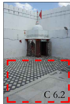
C 6.2 - Condition - Incompatible addition - Unlevelled Flooring - causing ingress of water - damage to floor
